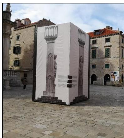
Orlando's staircase is in poor condition with significant structural damage. The Institute for Reconstruction has agreed to set up a protective skeleton around Orlando's staircase with the Croatian Restorers' Institute, and to conduct monitoring of the damage over two years, at
